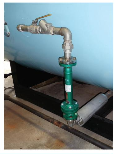
a hard and brittle calcite scale buildup on heat transfer surfaces of equipment and piping. Instead, the minerals push away and repel one another, at the molecular level, and precipitate out of solution in a softer suspended state commonly called aragonite, which will either flow right on through the plumbing system, or drop to a low point in water-using equipment where they can easily be purged through blow-down (draining).
