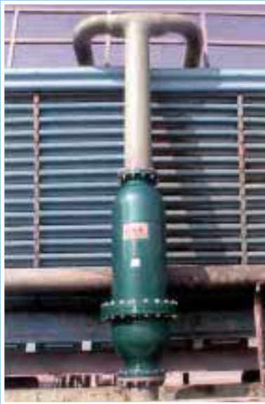
ACV-14-K-10 Installed on a 1,000 ton Cooling Tower
