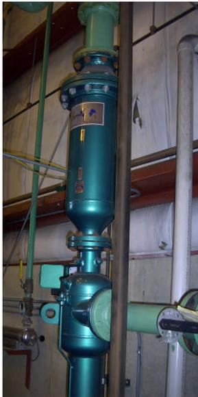
For years, chemicals have been the traditional and conventional method used to control these problems in heat-transfer equipment. Yet, when the Superior Water Conditioner<sup>®</sup> is used in conjunction with centrifugal separation and filtration equipment (Superior's "Environmentalist/Zero-Bleed 2000<sup>®</sup>"), no chemicals are needed and bleed requirements are totally eliminated.
