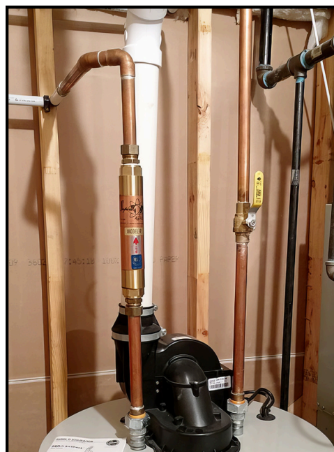
Superior unit installed on a standard water heater
